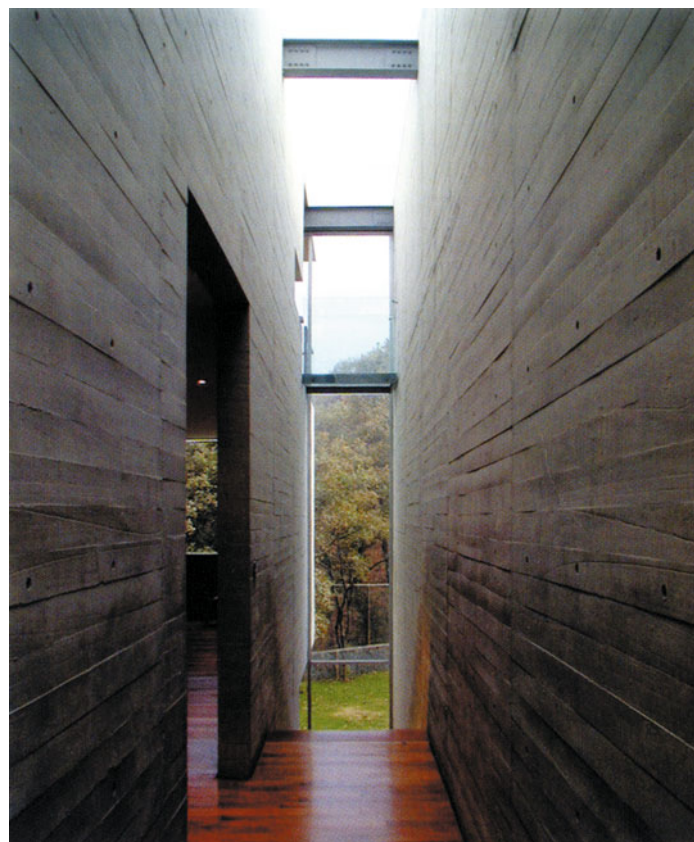
CASA F2. GROUND FLOOR LANDING AND STAIRWELL ON WEST SIDE OF THE HOUSE.
