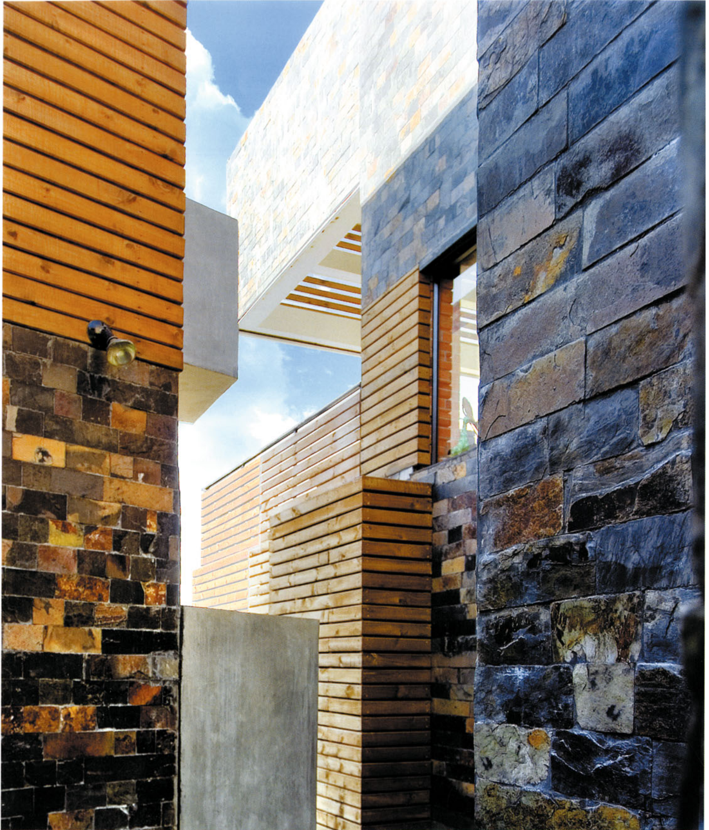
CASA JG. VIEW OF THE PASSAGE BETWEEN THE SOCIAL AND PRIVATE BLOCKS.
