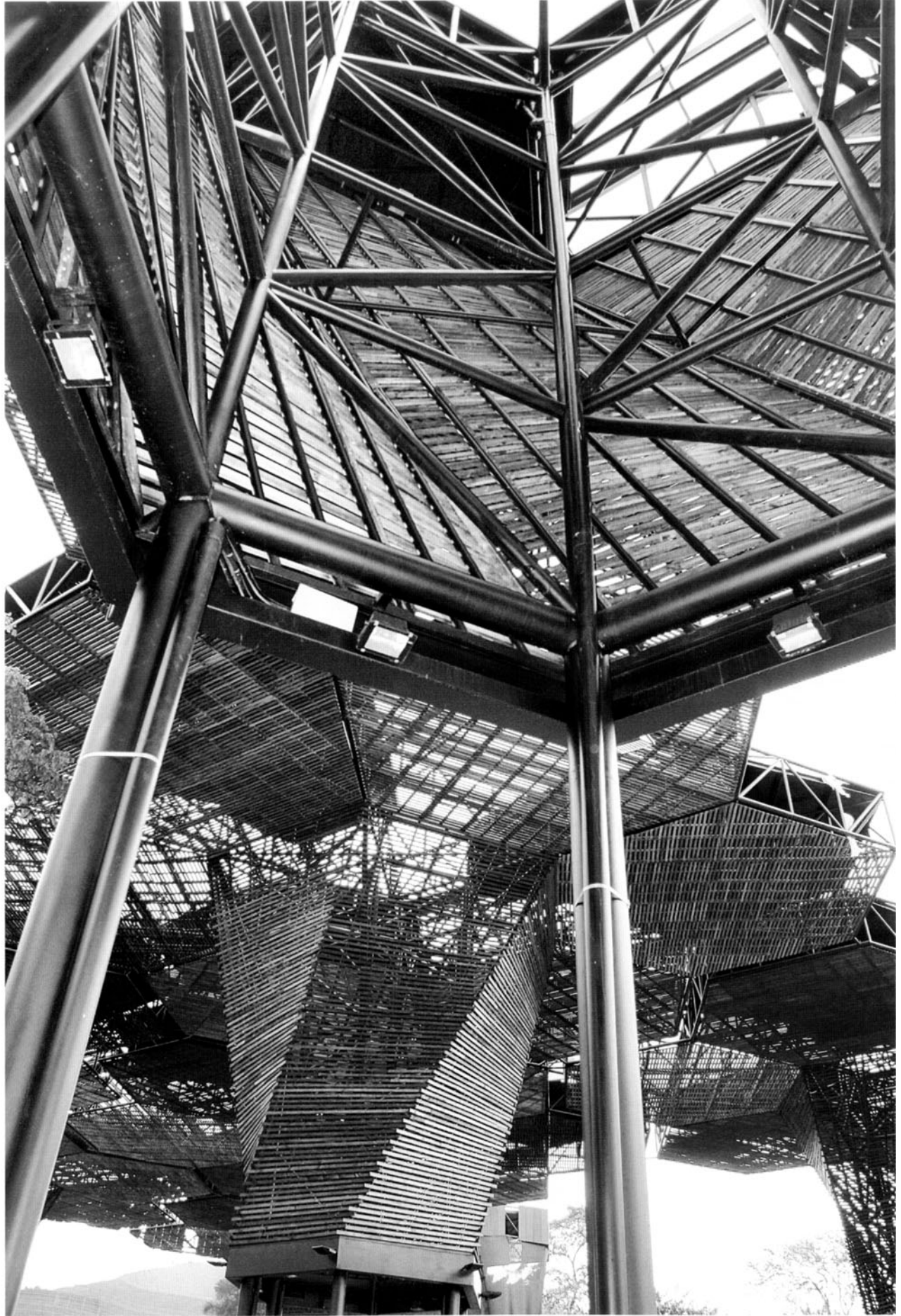
ORQUIDEORAMA. THE METAL STRUCTURE OF THE 'FLOWER-TREES'.
