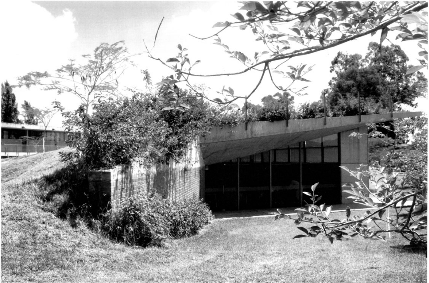
LICEO FRANCO-MEXICANO. VIEW OF THE RETAINING WALL AND THE TOPOGRAPHIC SOLUTION AT THE END OF THE ROW OF CLASSROOMS.
