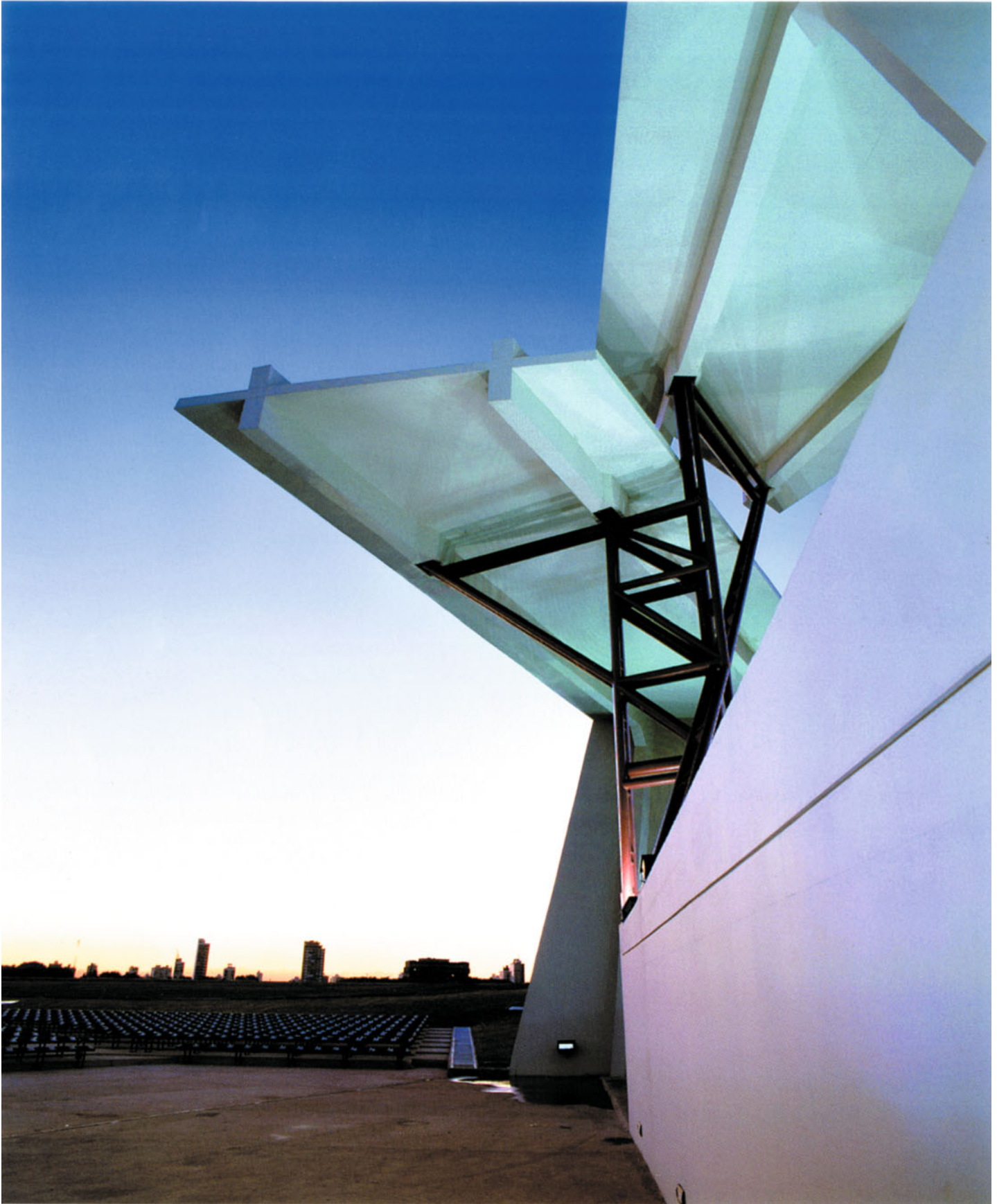
PASEO COSTA, ANFITEATRO COSTA. OUTDOOR THEATRE STAGE AND SITTING AREA WITH THE CITY IN THE BACKGROUND.
