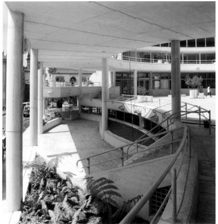
FONDO DE CULTURA ECONÓMICA. MAIN ACCESS SHOWING THE INTRICATE SOLUTION OF LEVELS AND CIRCULATIONS.
