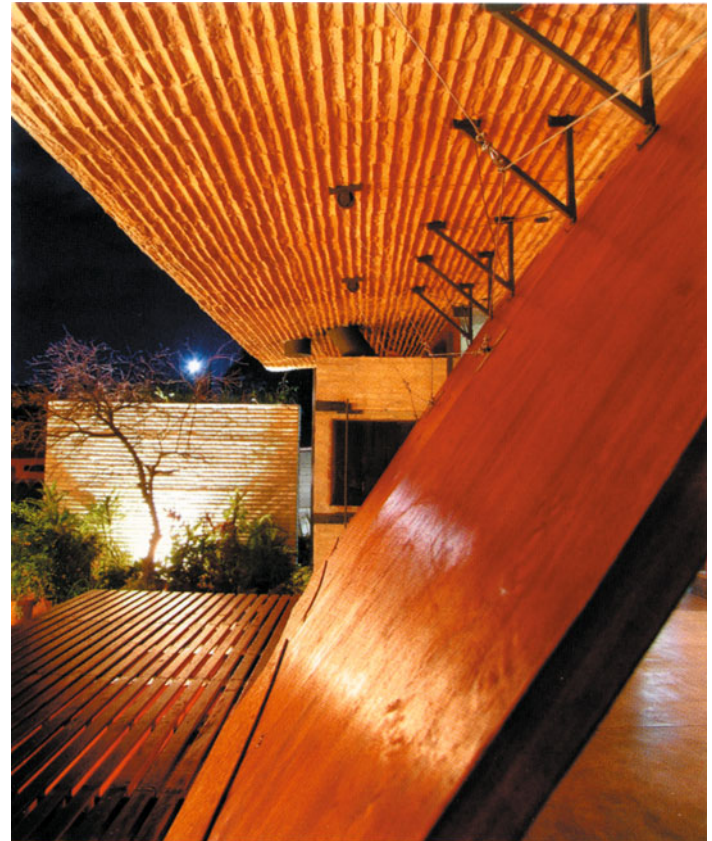
CASA ABU & FONT. VIEW OF THE MOVABLE WOOD PANELS AT THE REAR OF THE SOCIAL AREA OPENING ONTO TERRACE AND BACKYARD.
