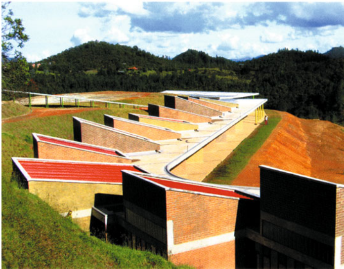
COLEGIO HONTANARES. VIEW OF THE UNDULATING ROW OF CLASSROOMS AND THE TERRACING SYSTEM.
