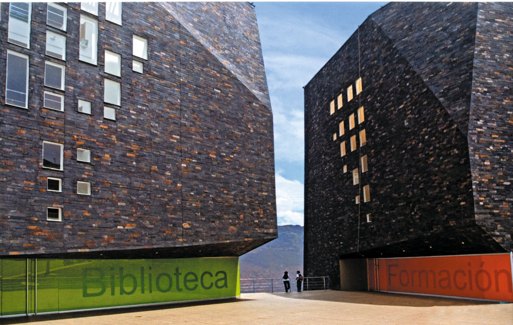
SANTO DOMINGO LIBRARY. VIEW FROM THE PLAZA.
