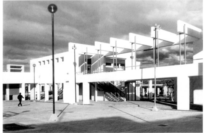
AVENIDA 24 DE MAYO. PEDESTRIAN BRIDGE AND ARCHWAY.
