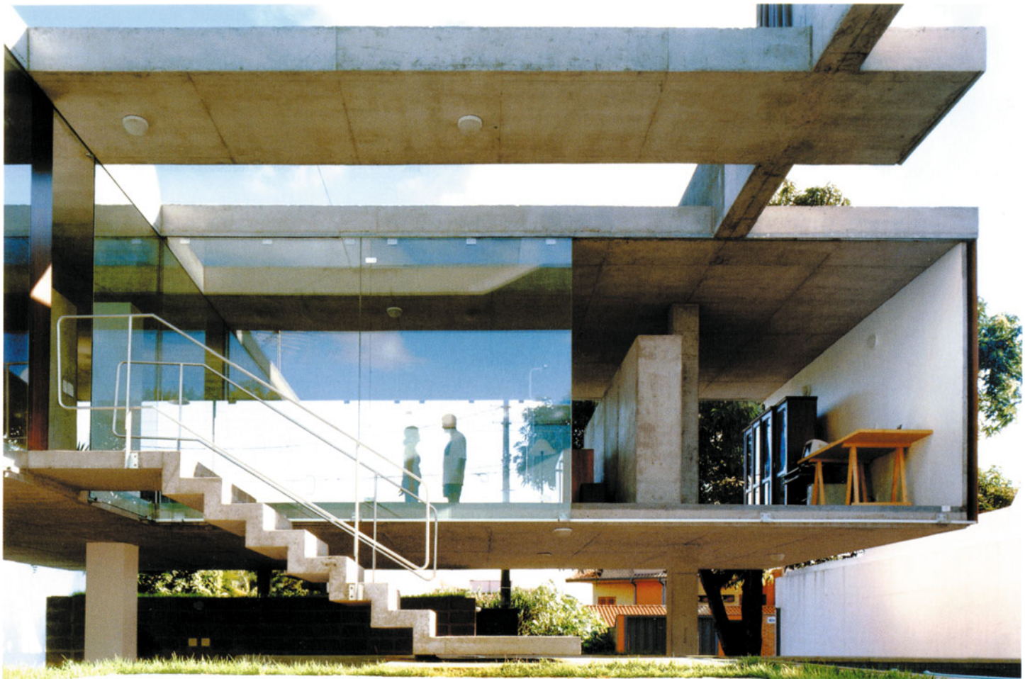
HOUSE IN RIBEIRÃO PRETO, BRAZIL, ANGELO BUCCI. VIEW OF THE COURTYARD, ACCESS AND THE SOCIAL AREA.
