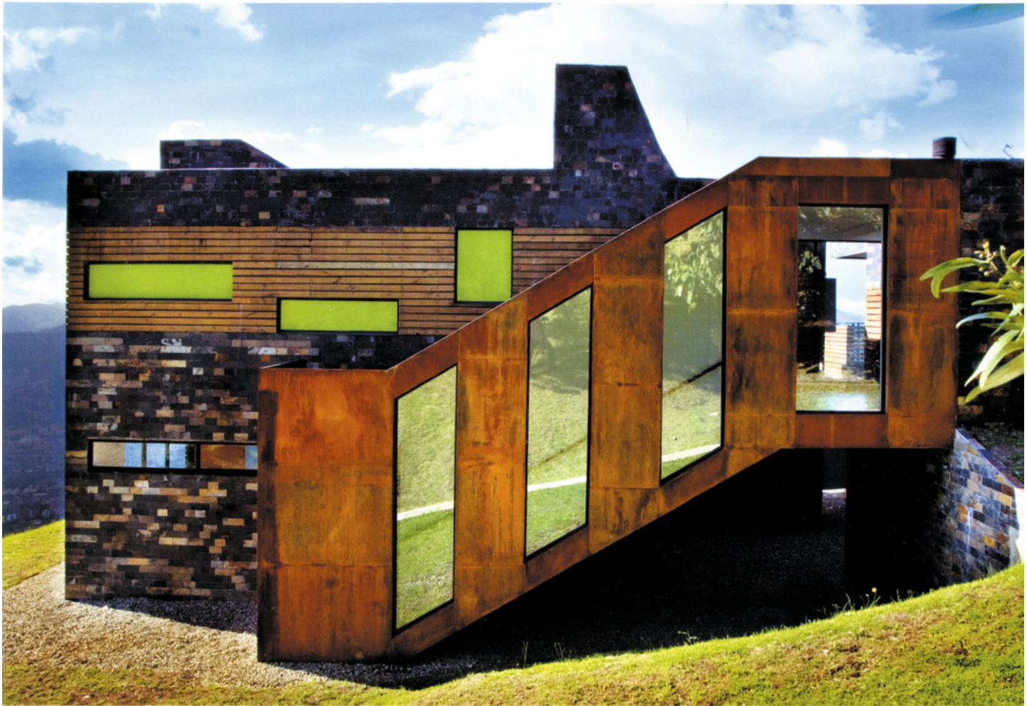
CASA JG. DETAIL OF THE BACK ELEVATION (EAST) SHOWING THE STAIRCASE TO THE CHILDREN'S QUARTERS.
