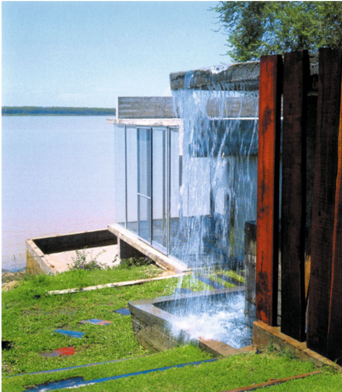
CASA EN LA BARANCA. VIEW OF THE ACCESS TO THE HOUSE WITH WATER CASCADING FROM THE SWIMMING POOL.
