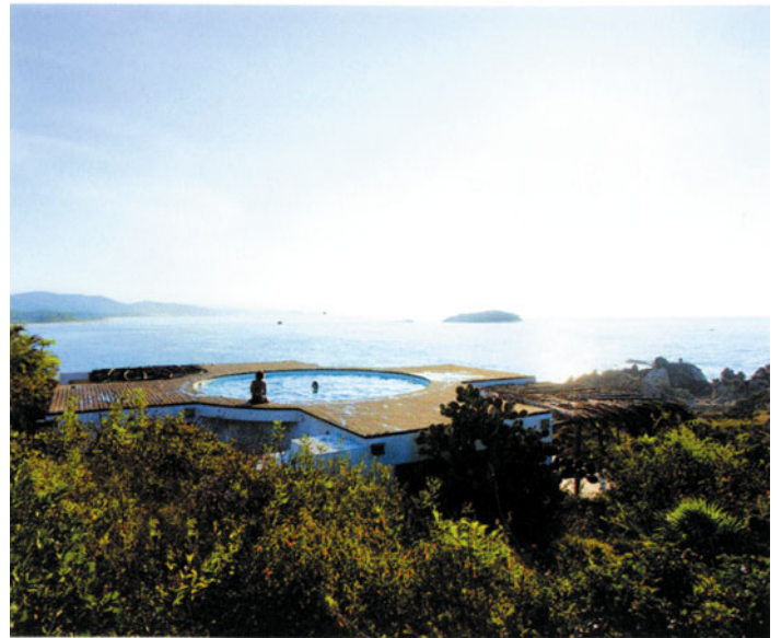
OBSERVATORY HOUSE. VIEW OF THE HOUSE WITH PACIFIC OCEAN IN THE BACKGROUND.
