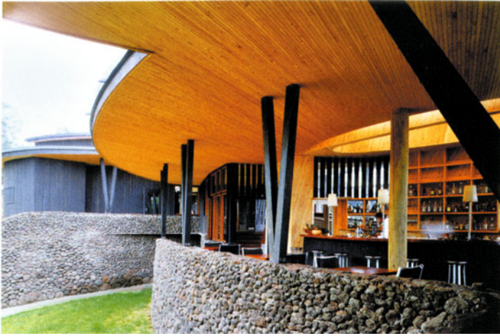
HOTEL EXPLORA. VIEW OF THE PERIPHERAL CIRCULATIONS UNDER THE CANOPY AND THE ARTICULATION OF MATERIALS ON THE EXTERIOR OF THE BUILDING.
