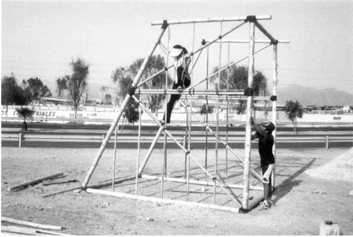
TEATINA-QUINCHA SHELTER. ERECTION OF BAMBOO STRUCTURE.
