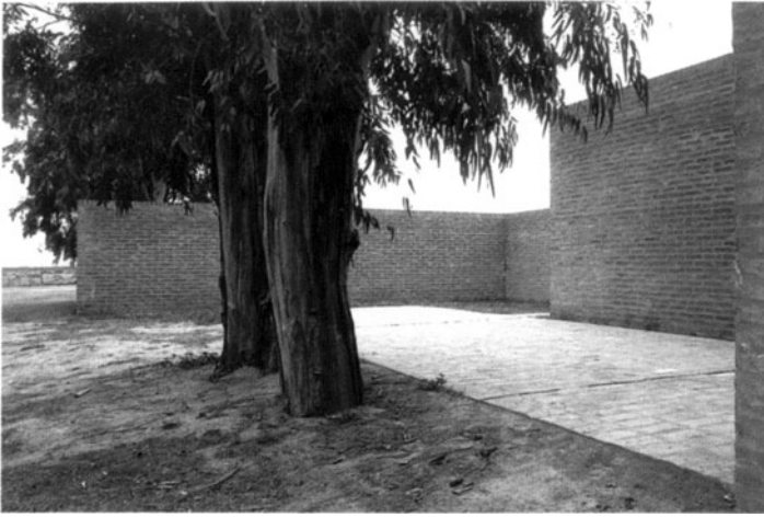
CASA DE CAMPO EN LA PLAYOSA. VIEW OF THE FORECOURT DEMARCATING THE APPROACH TO THE HOUSE.
