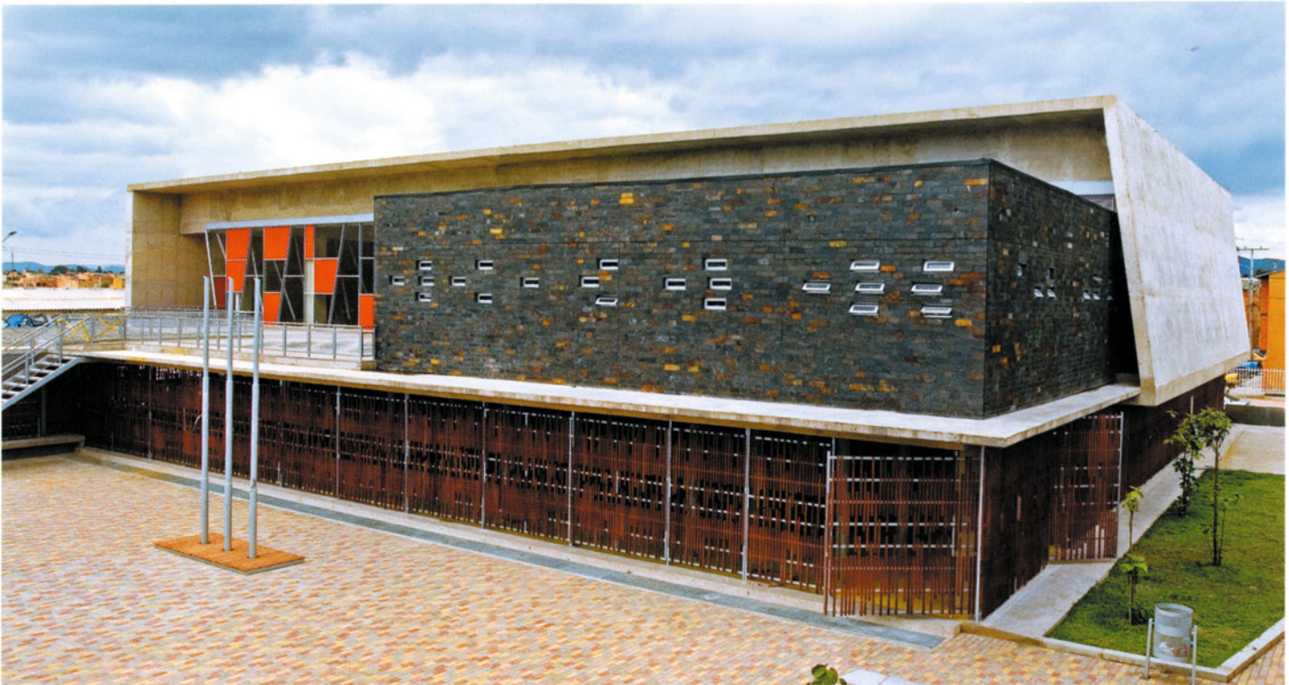
GERARDO MOLINA SCHOOL. AUDITORIUM AND MULTI-FUNCTIONAL ROOM.
