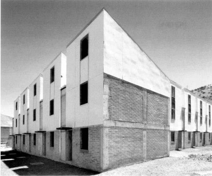
RENCA. LAST STAGES OF CONSTRUCTION.
