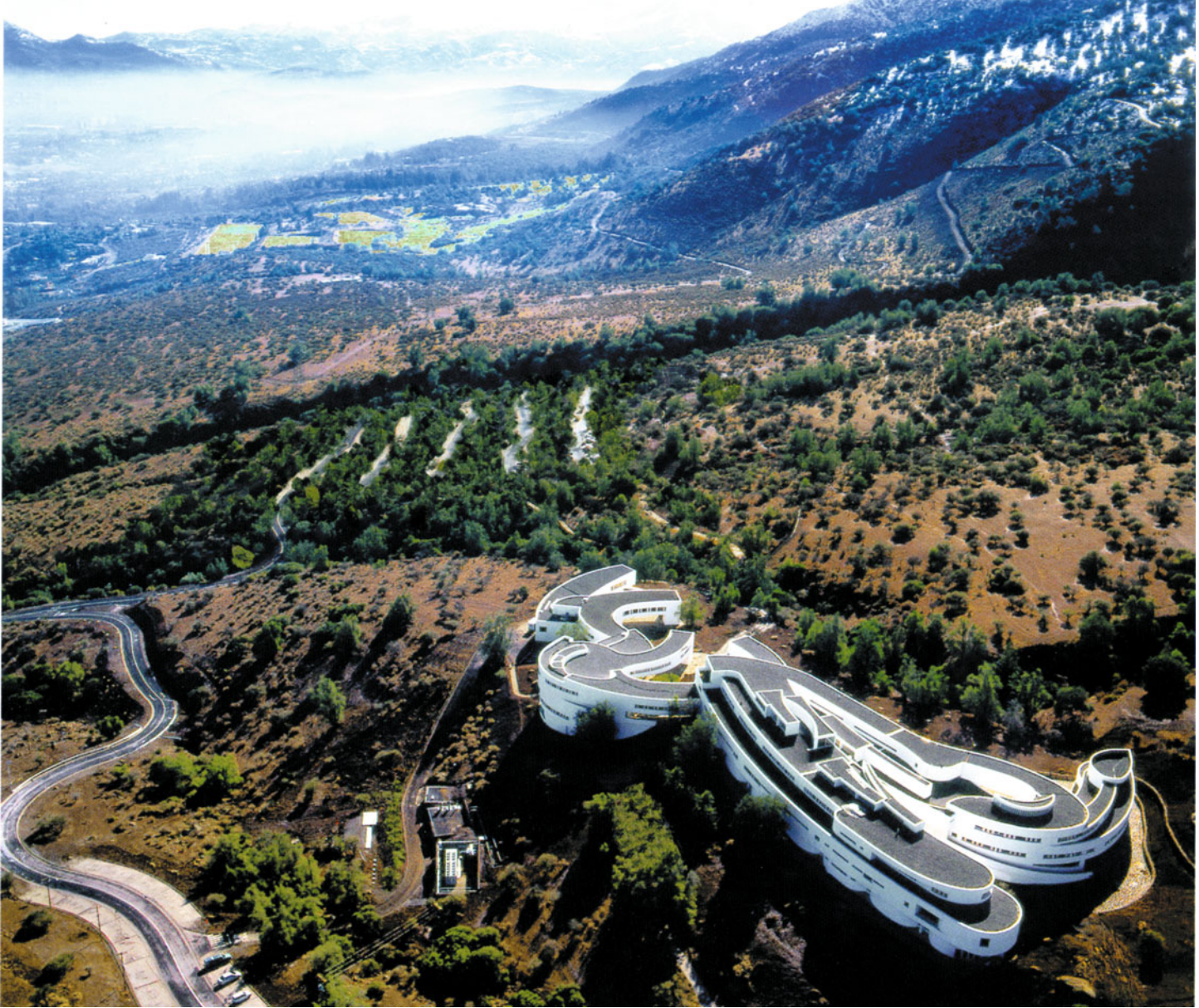
POSTGRADUATE BUILDING, UNIVERSIDAD ADOLFO IBAÑEZ. AERIAL VIEW OF THE BUILDING SHOWING ITS CORRESPONDENCE TO THE MORPHOLOGY OF THE CORDILLERA.
