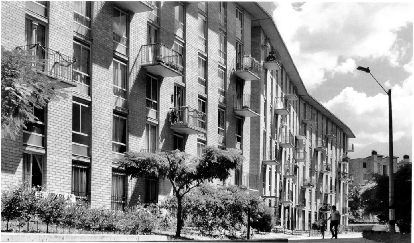
URBANIZACIÓN LA PLAYA. VIEW OF ONE OF THE BLOCKS FROM THE INTERNAL PUBLIC SPACE.
