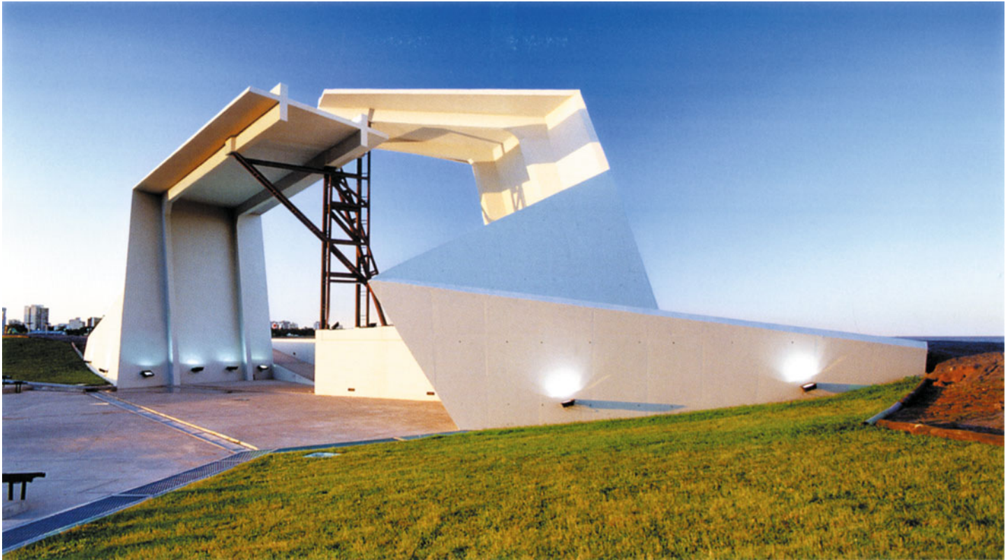
PASEO COSTA, ANFITEATRO COSTA, BUENOS AIRES, ARGENTINA, CLAUDIO VEKSTEIN. OUTDOOR THEATRE STAGE AND ACOUSTIC SHELL.
